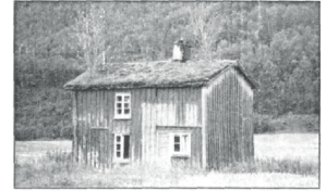
Fig. 2. House roofed with sod in Norway. Note the two trees that have taken root in the shallow soil. [OSmundson 121]
